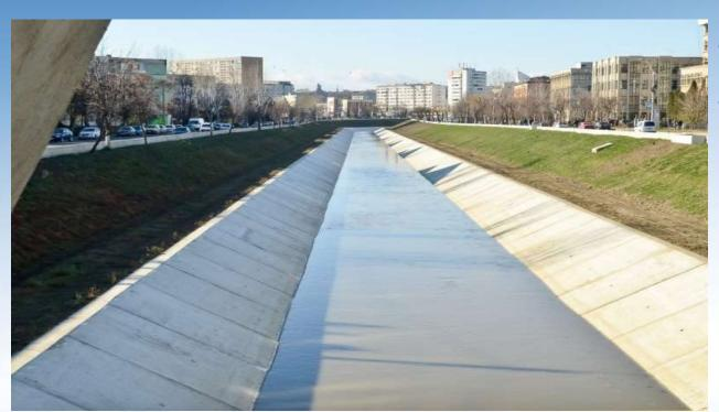
Bahlui river has been transformed by regularization and restoring the banks.
